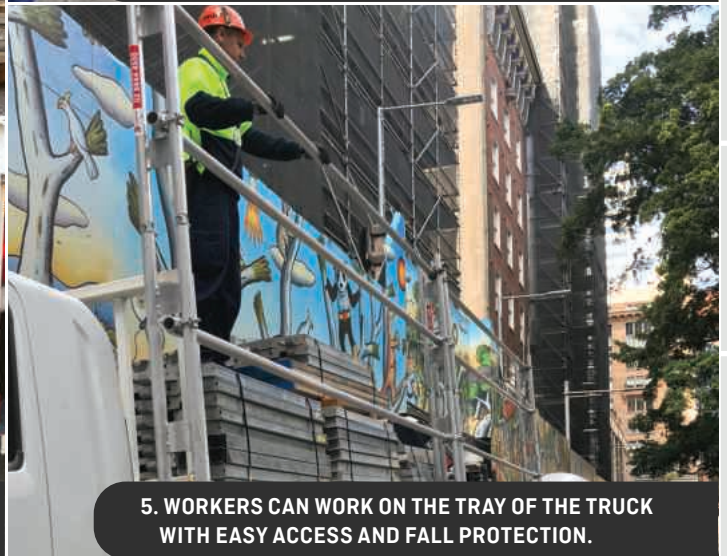
4. ACCESS PLATFORM IS PLACED ON THE TRAY OF THE TRUCK FOR ACCESS.
