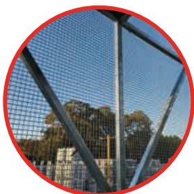
25mm x 25mm Mesh Encapsulation
