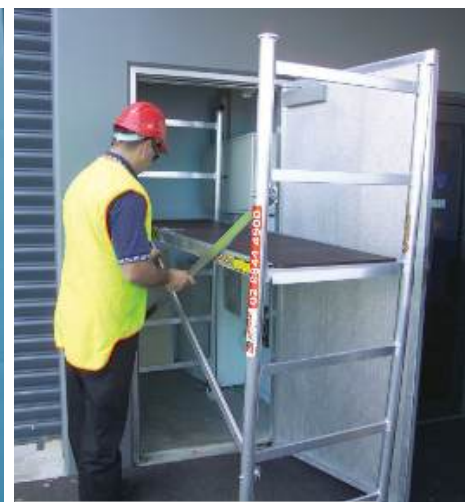
Standard Scaffold Fits Through Doorways
